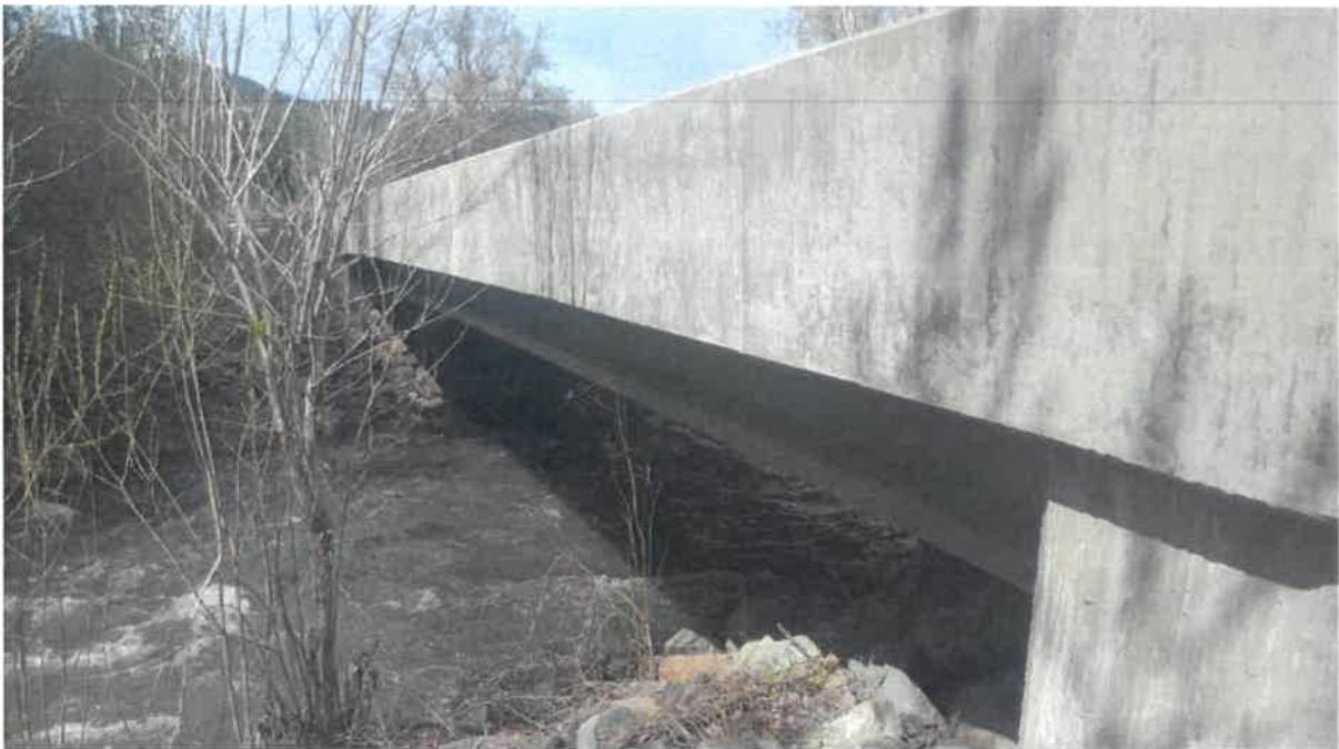
Photograph 12 – S Side of Burke Road Bridge Over Swauk Creek
