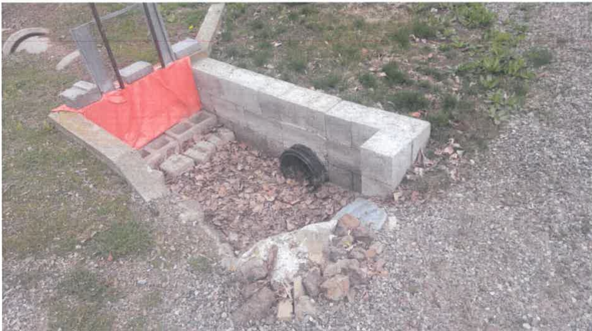
Photograph 10 – Flow Control Structure on East Canal/Pipeline N Side of Burke Road
