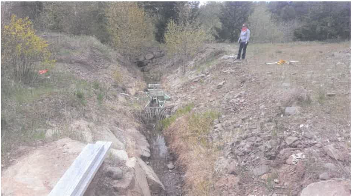
Photograph 2 – Fish Screen and Irrigation Canal from Diversion Structure
