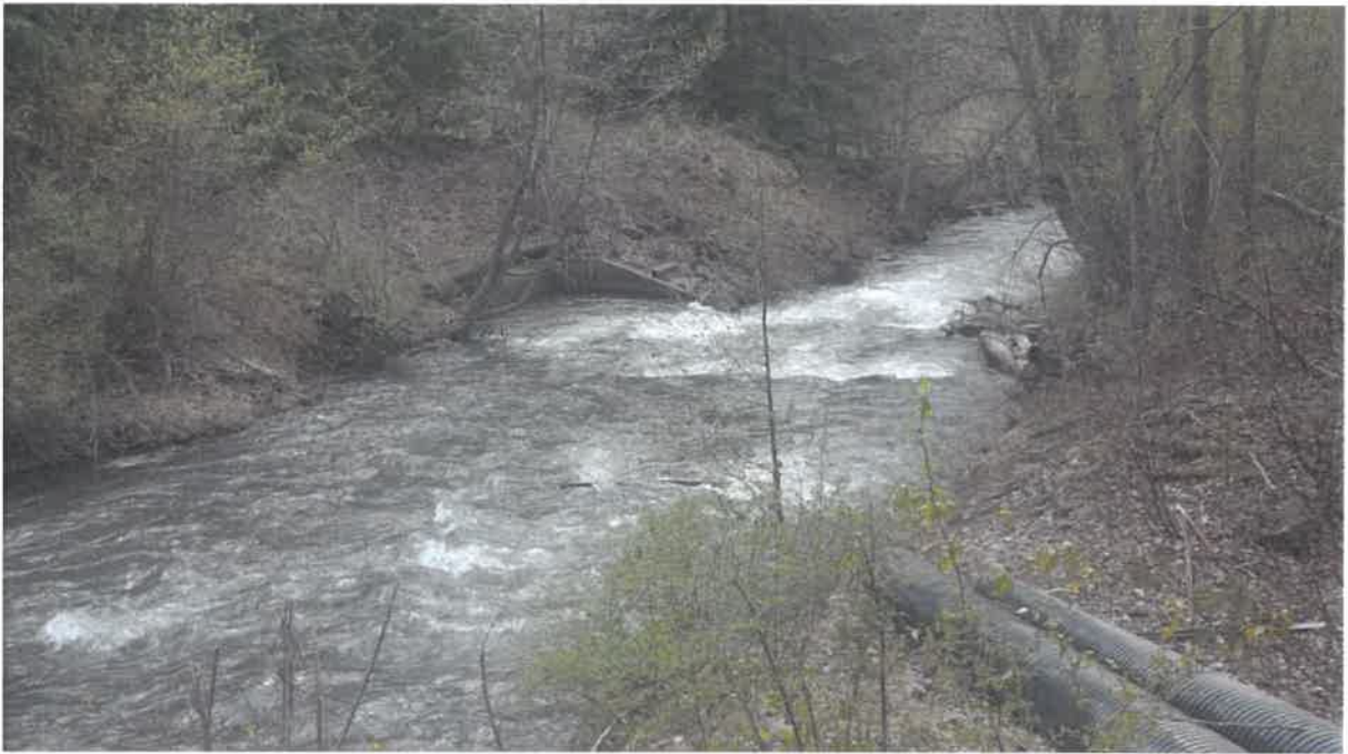
Photograph 7 – Downstream Irrigation Diversion Structure
