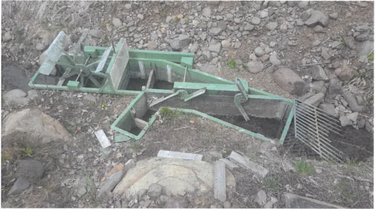
Photograph 3 – Fish Screen with Paddle Wheel
