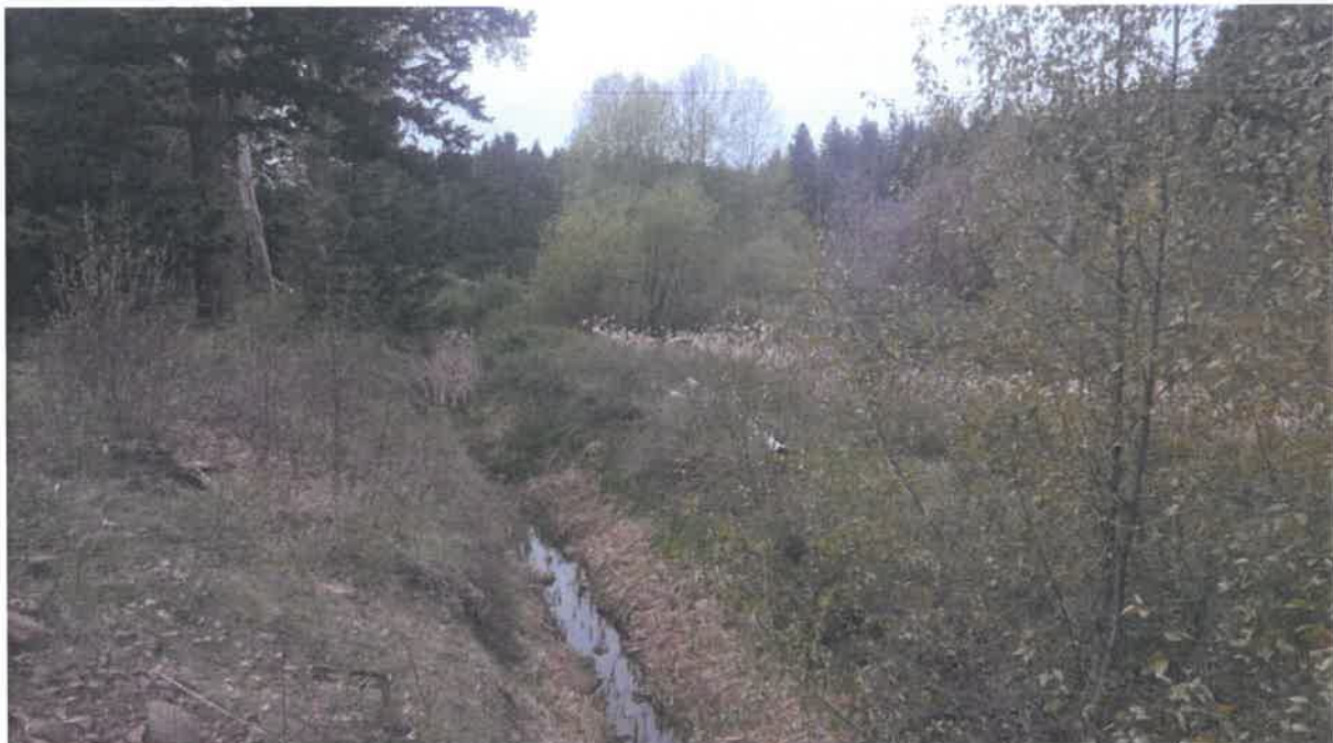
Photograph 6 – Irrigation Canal Downstream of Fish Screen on West Side of Creek
